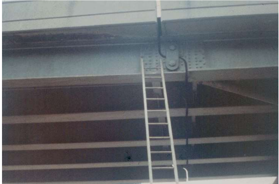
Figure 10.7.16 Multi-girder Bridge with Pin-and-Hanger Assemblies
