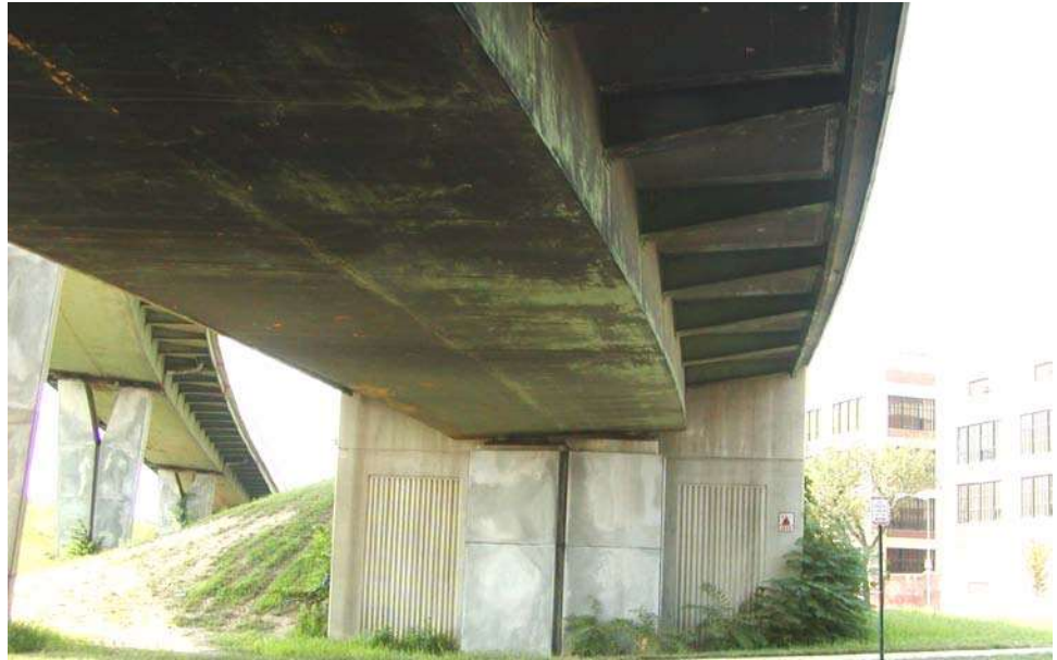
Figure 10.3.12 Non-Redundant Box Girder Bridges
