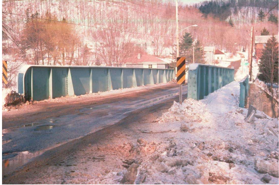
Figure 10.2.2 Through Girder Bridge
