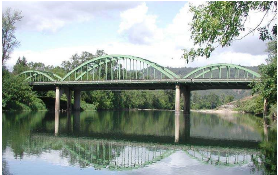
Figure 10.5.14 Three-Span Tied Arch Bridge
