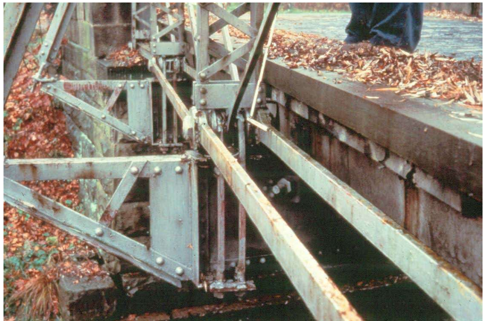
Figure 10.4.45 Bottom Chord with Eyebars
