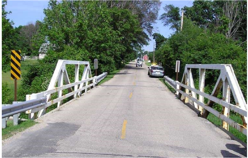
Figure 10.4.4 Pony Truss
