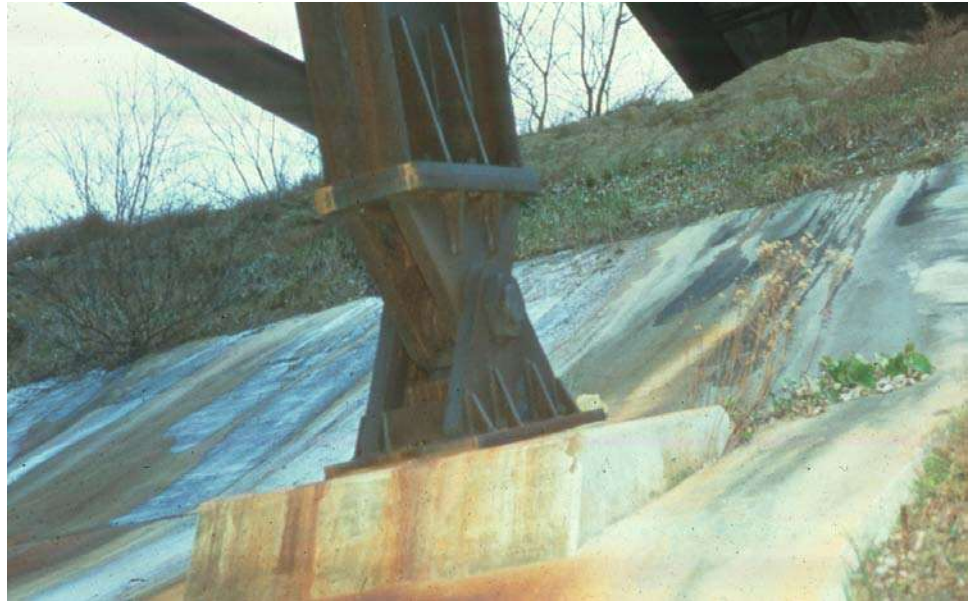
Figure 10.6.13 Bearing Area of a Two Frame Bridge
