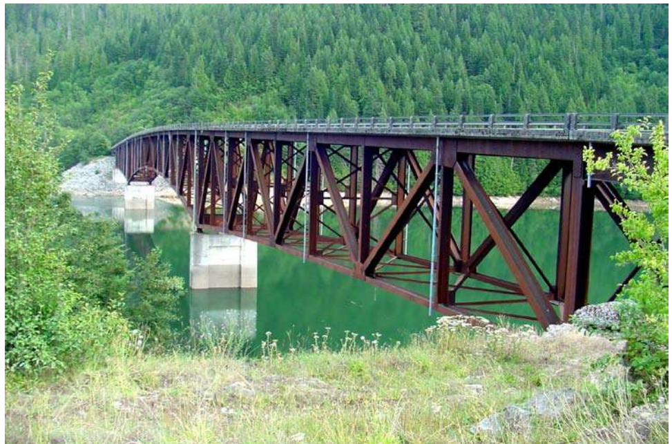
Figure 10.4.5 Deck Truss
