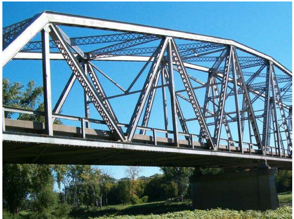
Figure 10.8.1 Steel Truss Superstructure with Gusset Plates
