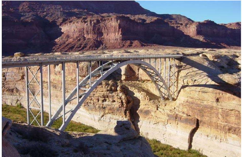
Figure 10.5.1 Deck Arch Bridge
