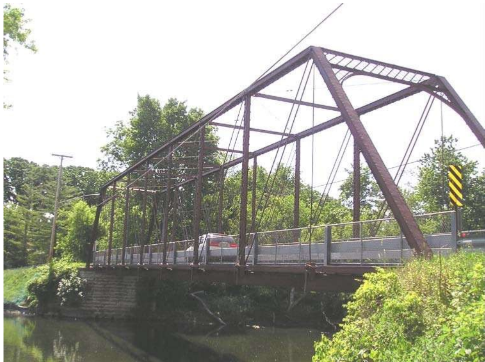
Figure 10.4.11 Single (Simple) Span Through Truss
