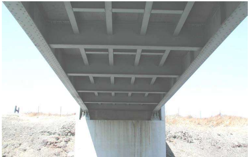
Figure 10.2.6 Two-Girder Bridge with Girder-Floorbeam-Stringer System
