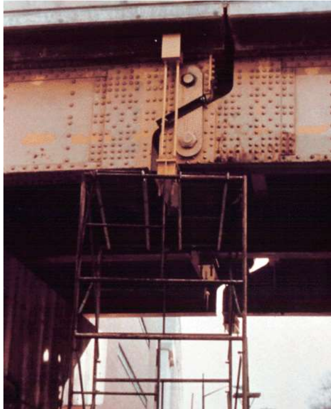
Figure 10.7.18 Alternate Hanger Link Retaining System
