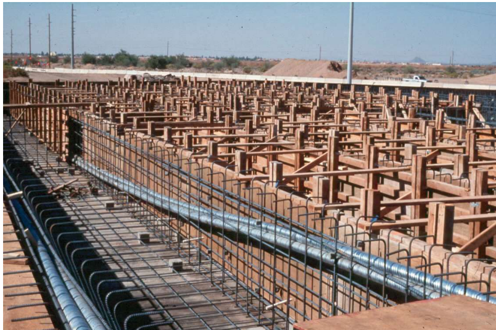
Figure 9.11.41 Post-tensioning Tendon Duct
