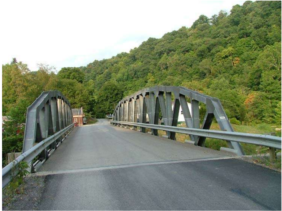
Figure 10.4.10 Single (Simple) Span Camel Back Pratt Truss
