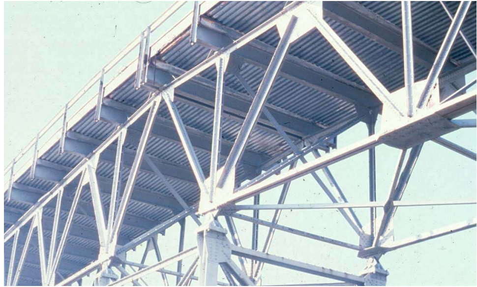
Figure 10.4.32 Floorbeam Floor System
