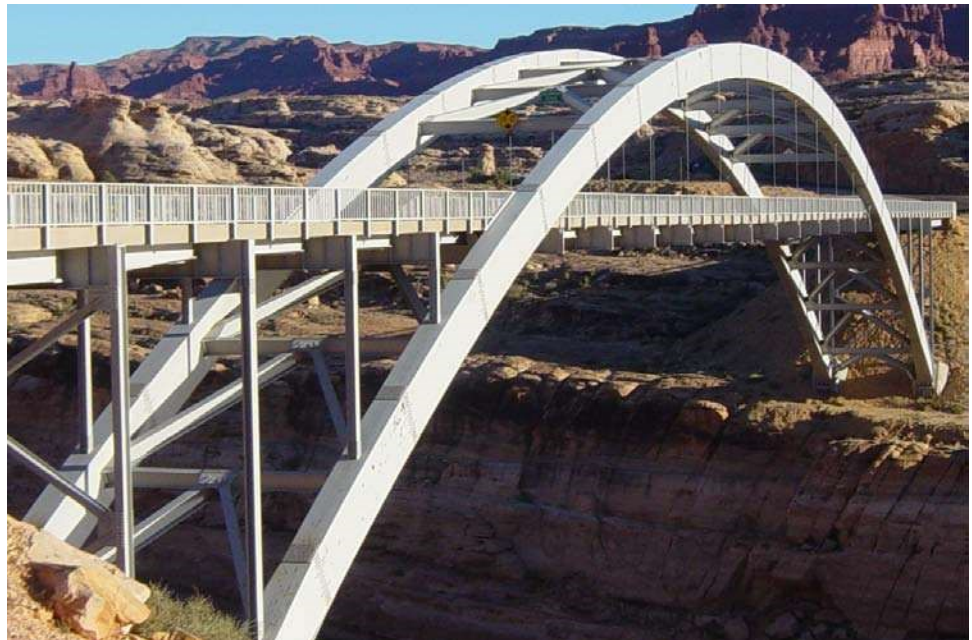
Figure 10.5.2 Through Arch Bridge
