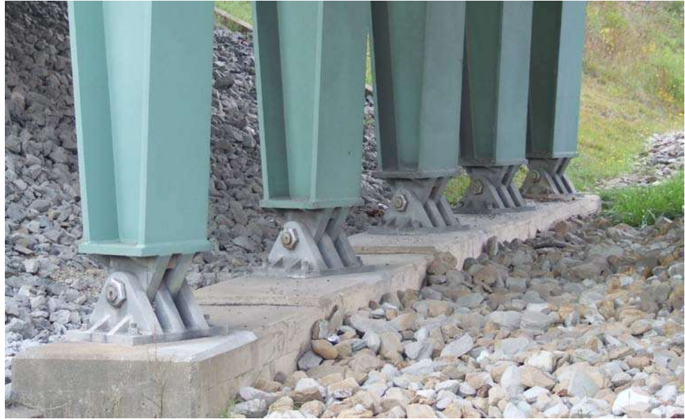
Figure 10.6.5 Bearings
