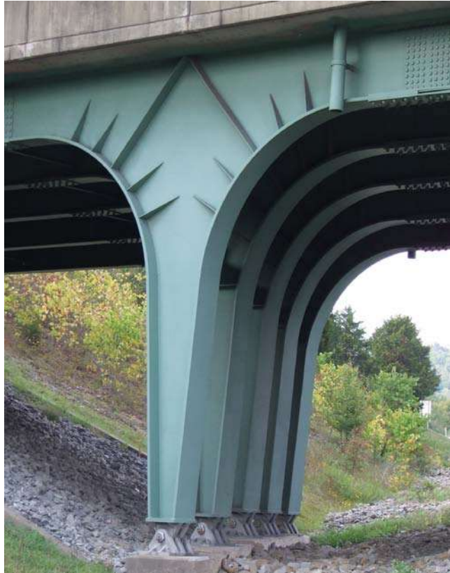
Figure 10.6.2 Typical Rigid Frame Constructed of Multiple Frames
