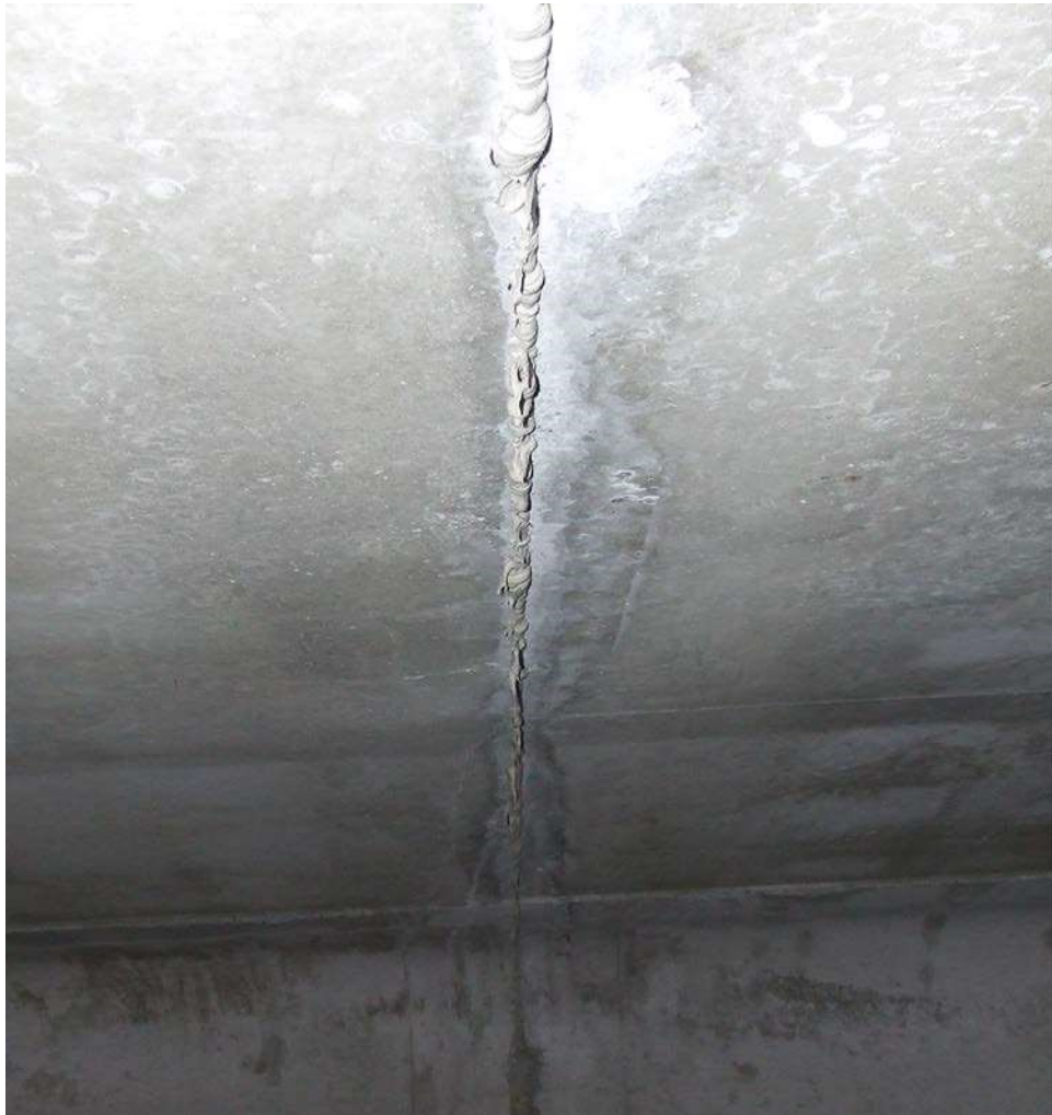
Figure 9.11.46 Close-up View of Box Girder Joint
