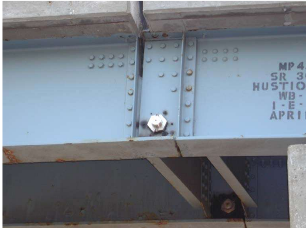
Figure 10.7.2 Single Pin with Riveted Pin Plate
