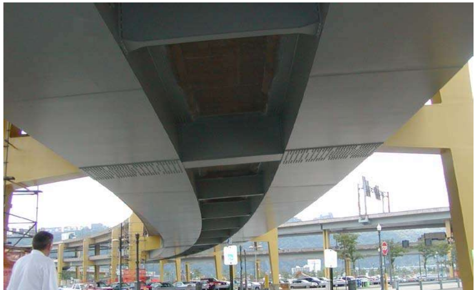
Figure 10.3.4 Spread Box Girders
