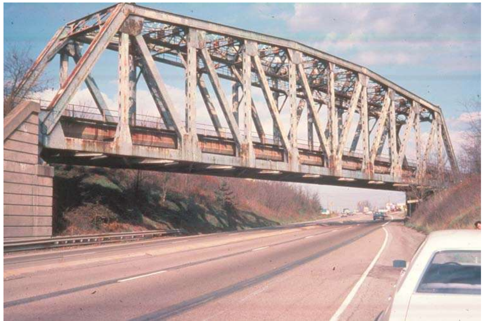
Figure 10.4.1 Simple Span Truss
