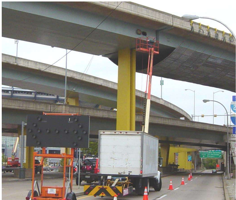
Figure 10.3.7 Box Girder Access Door
