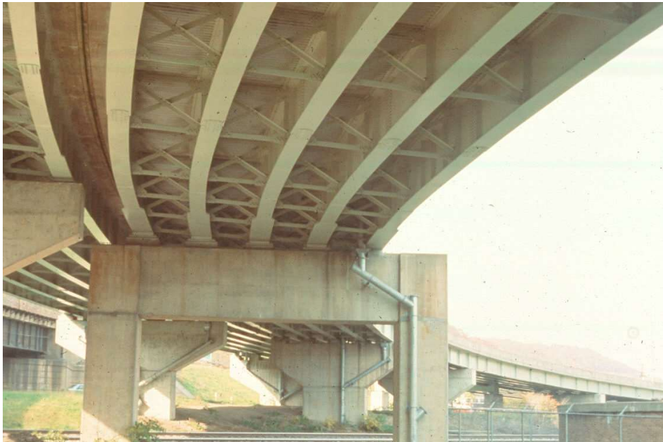
Figure 10.1.8 Curved Fabricated Multi-girder Bridge
