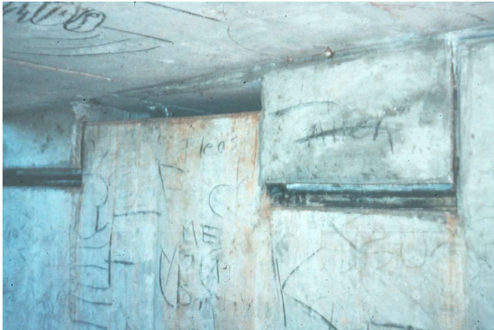
Figure 9.11.28 Bearing Area of a Box Girder Bridge
