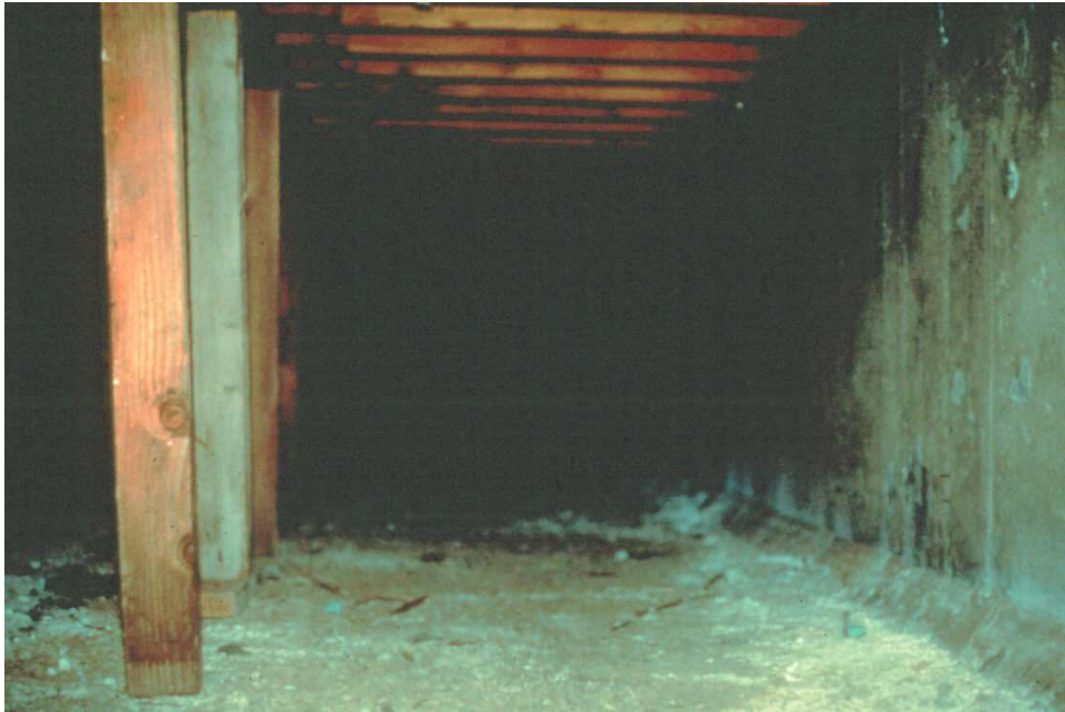
Figure 9.11.42 Interior Formwork Left in Place
