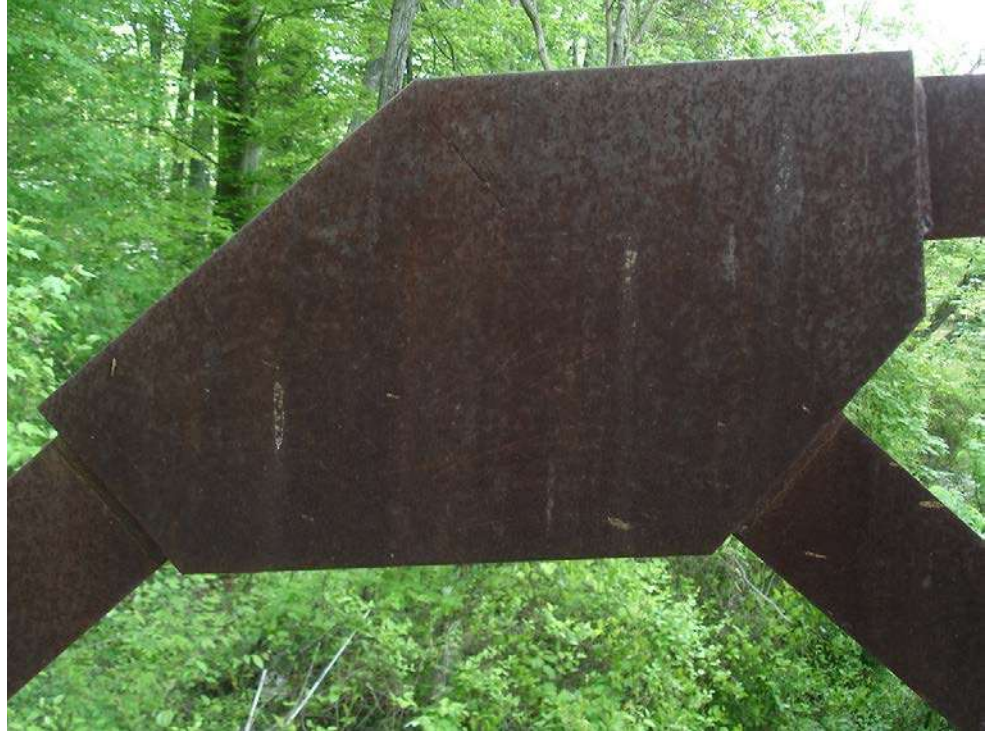
Figure 10.8.4 Steel Gusset Plate with Welded Connections
