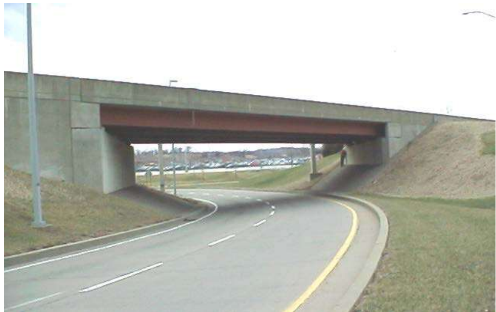
Figure 10.1.6 Single Span Fabricated Multi-girder Bridge
