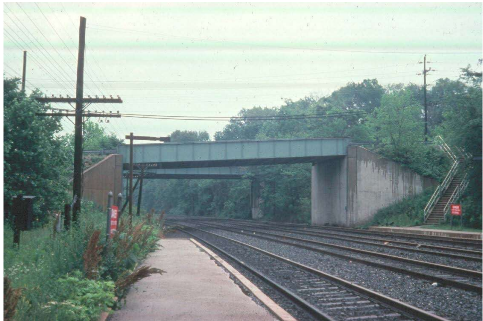
Figure 10.2.3 Through Girder Bridge with Limited Underclearance
