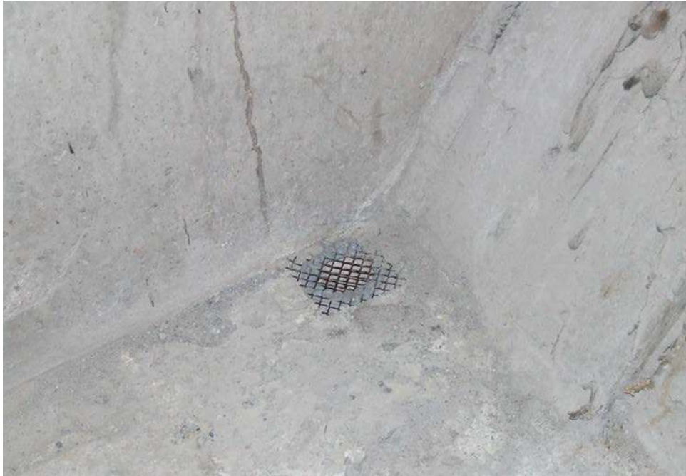
Figure 9.11.37 Concrete Box Girder Drain Hole with Screen
