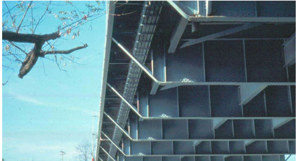
Figure 10.5.18 Floor System on a Through Arch
