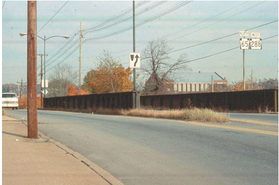
Figure 10.2.4 Through Girder Bridge with Three Girders
