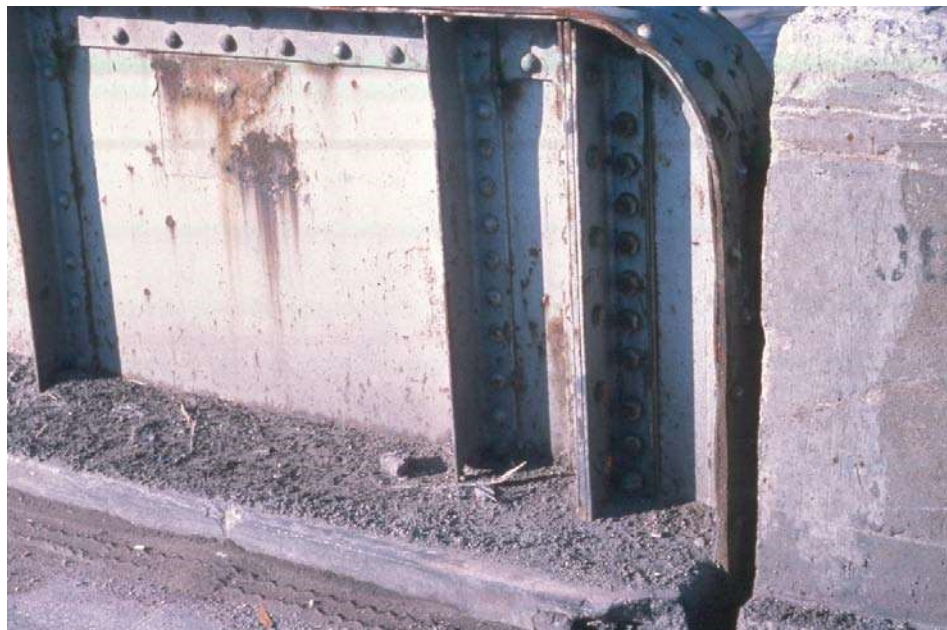
Figure 10.2.12 Web Area Near Support on a Through Girder Bridge
