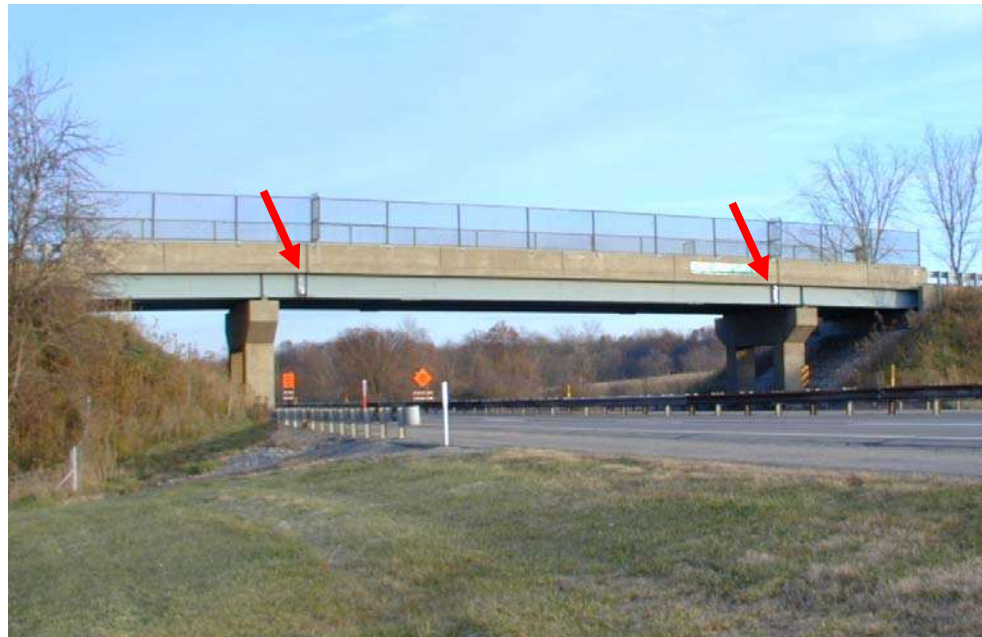
Figure 10.7.3 Pin-and-Hanger Assembly Locations Relative to Piers
