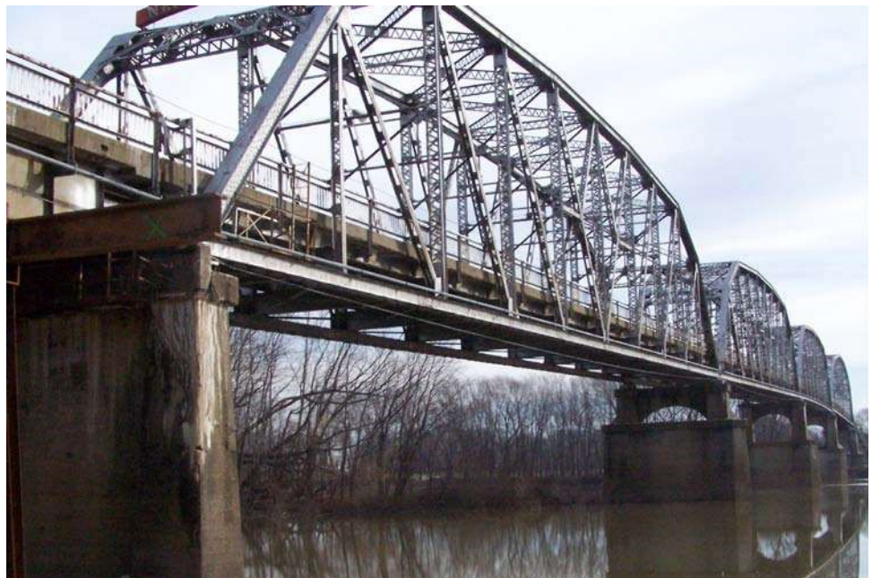
Figure 10.4.13 Multiple Span Through Truss
