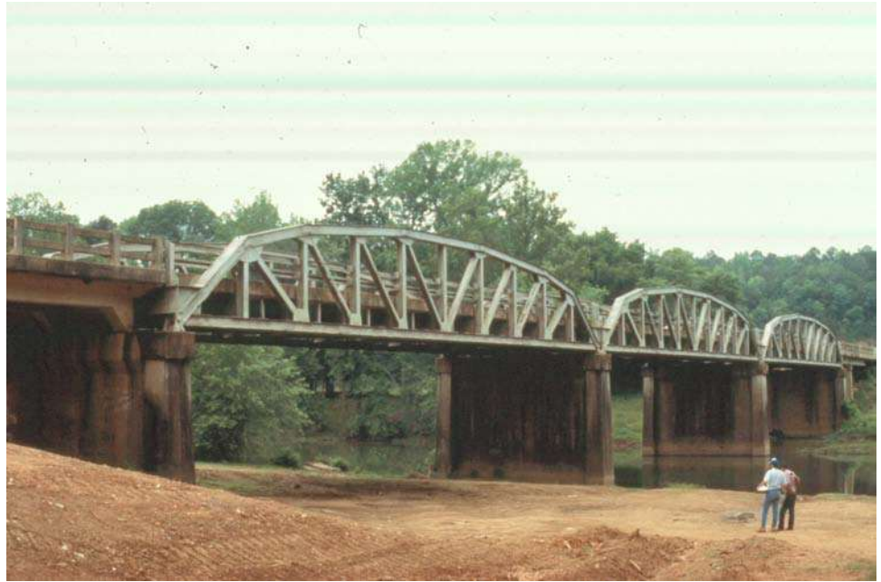
Figure 10.4.12 Multiple Span Pony Truss
