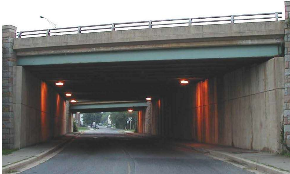
Figure 10.1.1 Simple Span Rolled Multi-Beam Bridge
