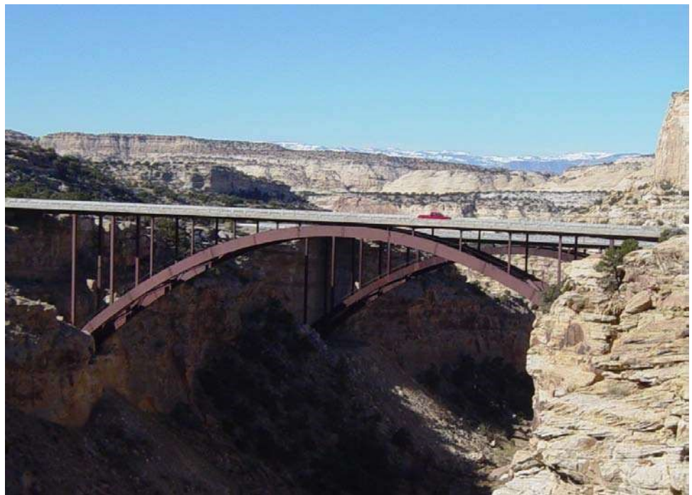
Figure 10.5.5 Solid Ribbed Deck Arch
