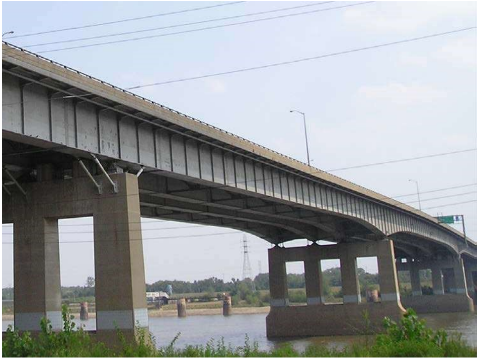
Figure 10.1.7 Continuous Span Fabricated Multi-girder Bridge
