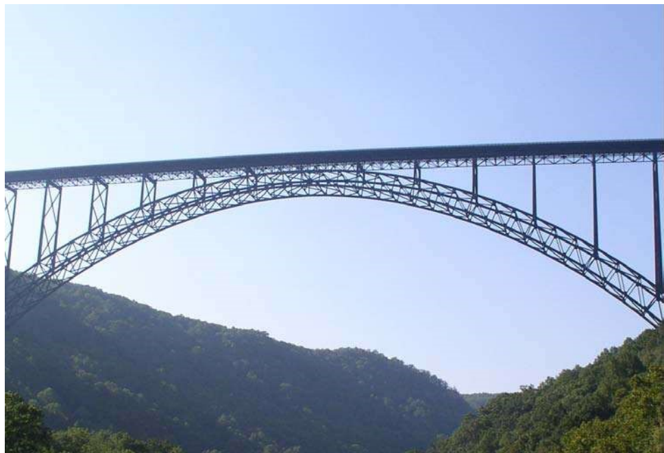
Figure 10.4.7 Deck Arch Bridge with Stiffening Truss
