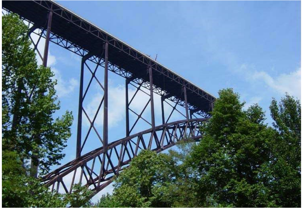
Figure 10.5.20 Braced Rib Deck Arch Showing Spandrel Columns
