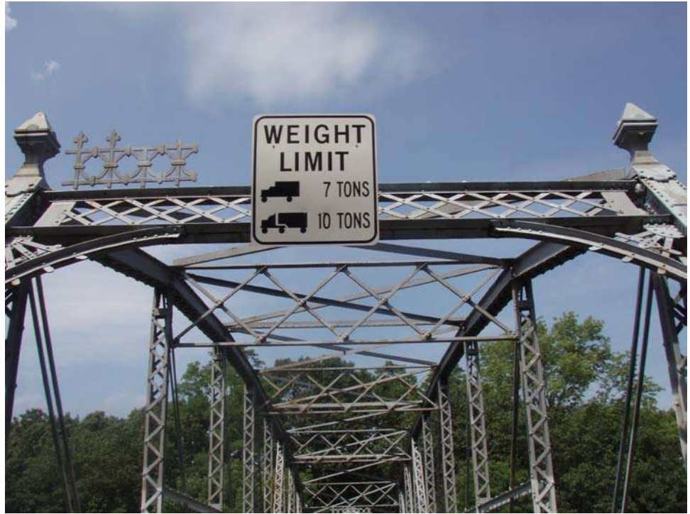
Figure 10.4.38 Portal Bracing with Attached Load Posting Sign
