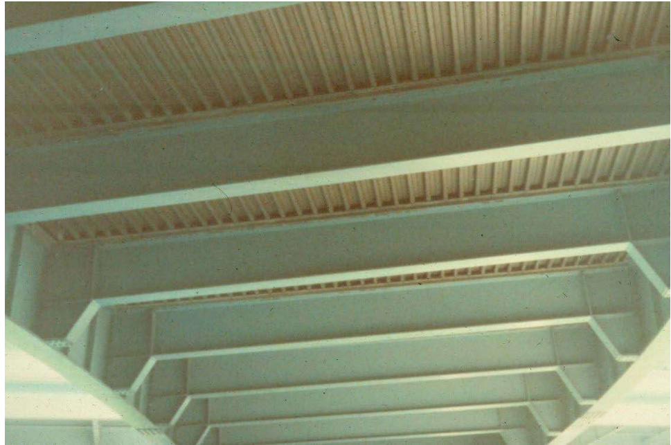
Figure 10.2.5 Two-Girder Bridge with Girder-Floorbeam System
