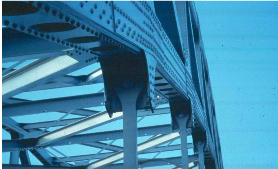
Figure 10.5.21 Hanger Connection on a Through Arch
