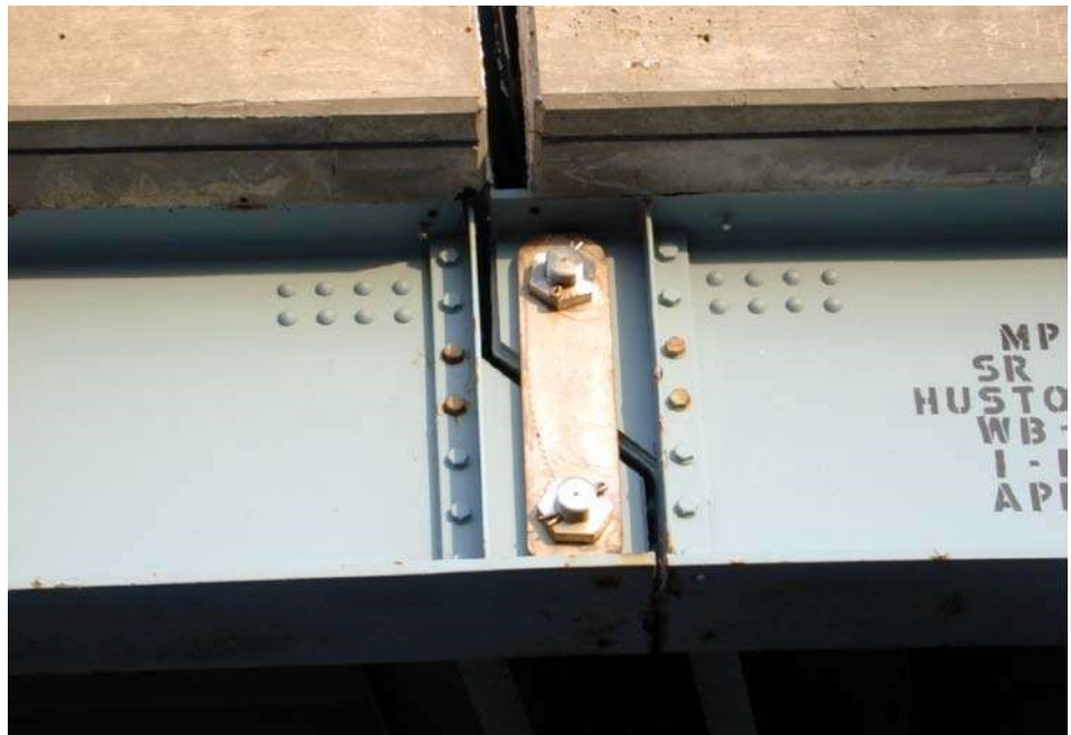
Figure 10.7.26 Stainless Steel Pin-and-Hanger Assembly
