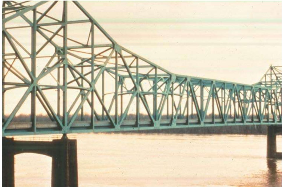
Figure 10.4.16 Cantilever Through Truss
