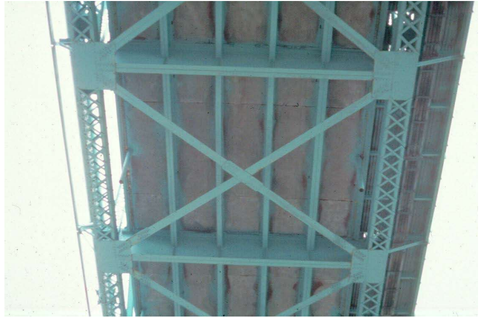
Figure 10.4.34 Lower Lateral Bracing
