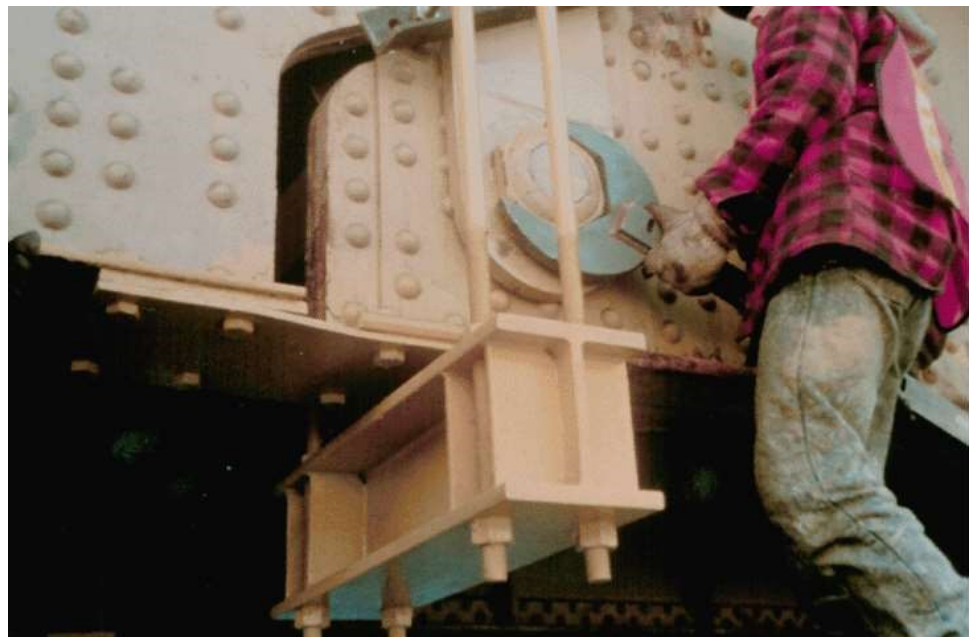
Figure 10.7.9 Retaining Nut
