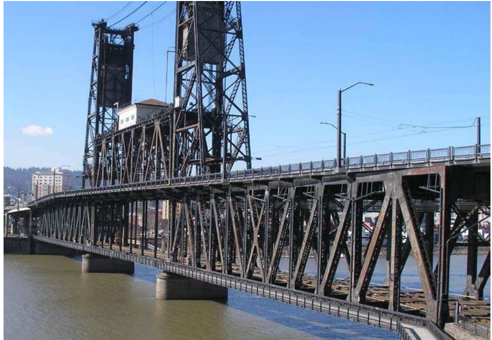
Figure 10.4.8 Vertical Lift Bridge
