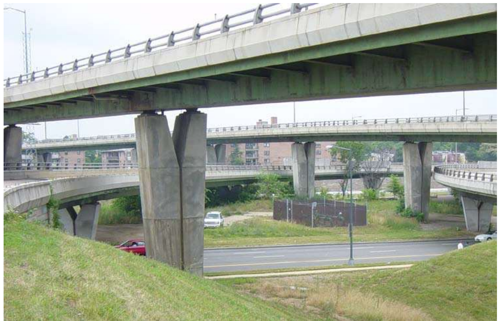
Figure 10.3.11 Continuous Box Girders
