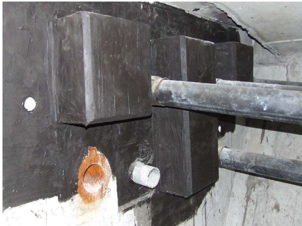
Figure 9.11.48 Box Girder Interior Diaphragm and Post-Tensioning Ducts
