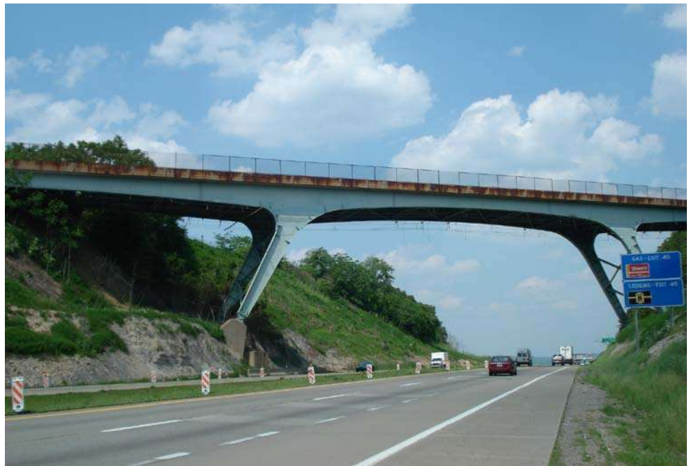
Figure 10.6.1 Typical Rigid K-frame Constructed of Two Frames
