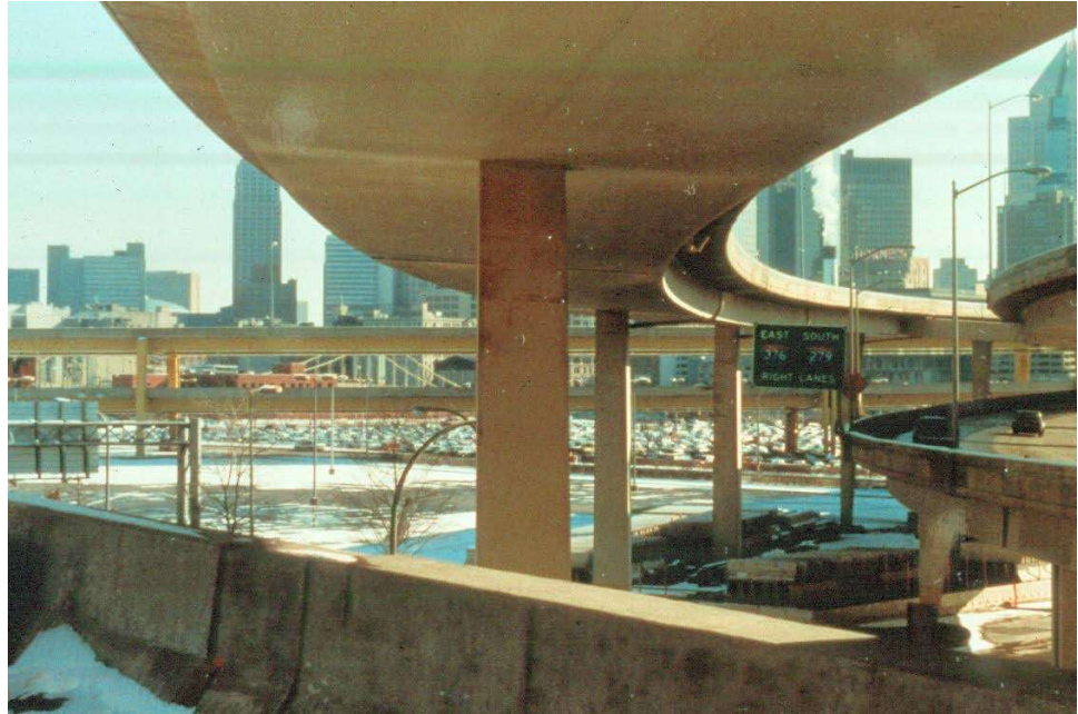
Figure 10.3.3 Box Girders With Multiple Interior Webs
