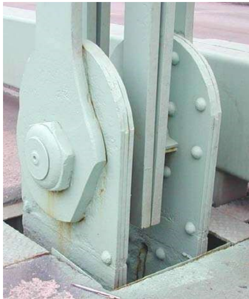
Figure 10.4.17 Pin-and-Hanger Assembly for Cantilevered Truss
