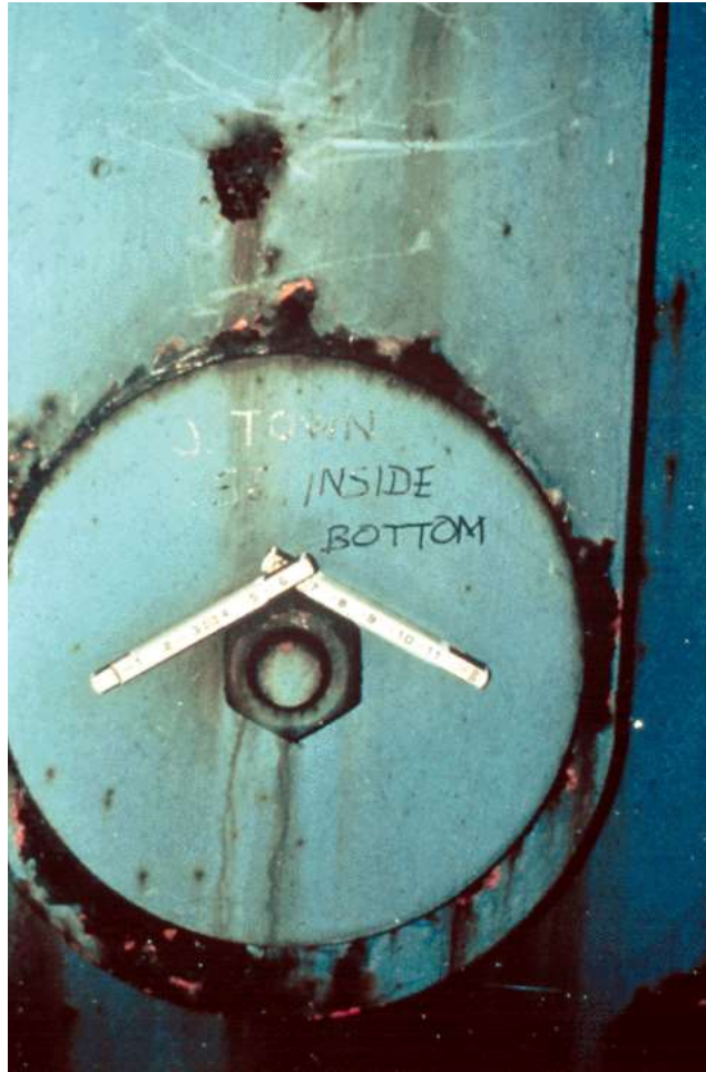
Figure 10.7.8 Pin Cap, Through Bolt and Nut
