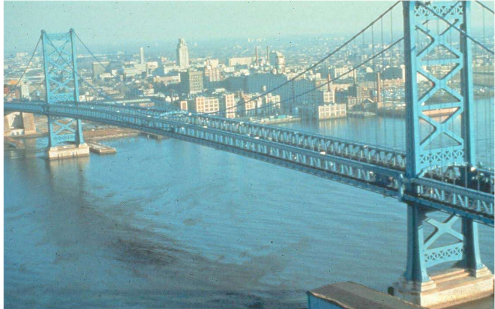
Figure 10.4.6 Suspension Bridge with Stiffening Truss
