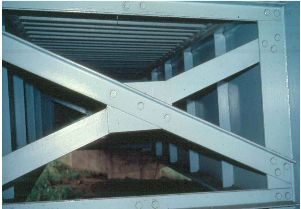
Figure 10.1.22 Intermediate Diaphragm
