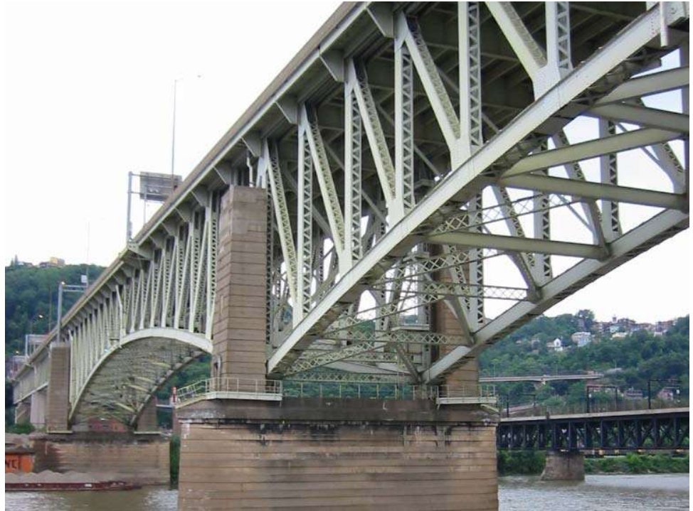
Figure 10.5.23 Bracing Members in Deck Arch Bridge
