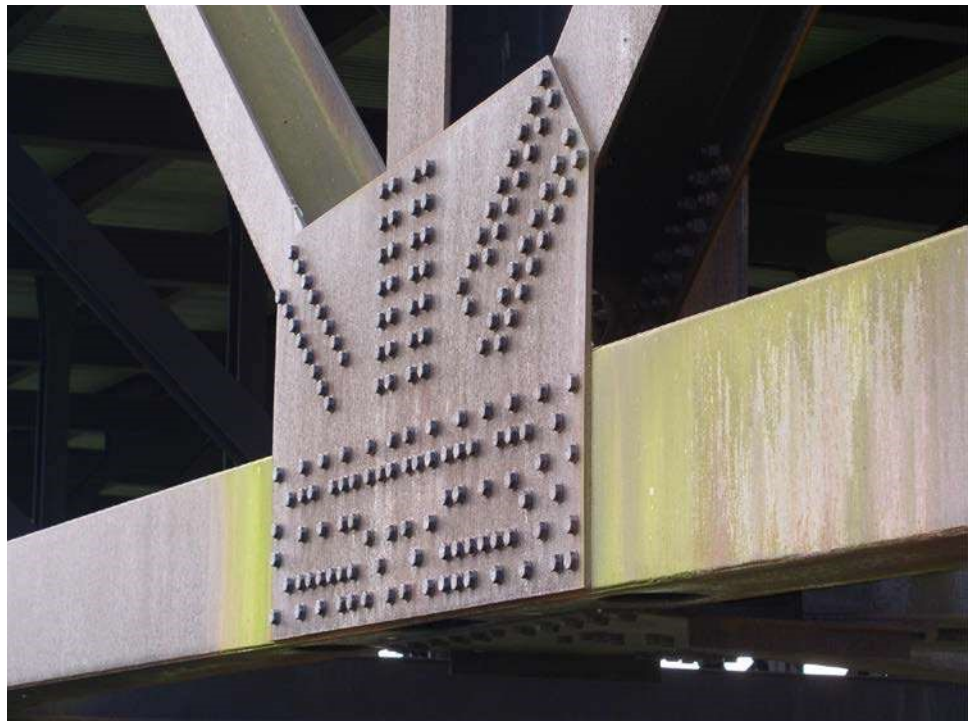
Figure 10.8.8 Gusset Plate Connecting Primary Load-Carrying Truss Members
