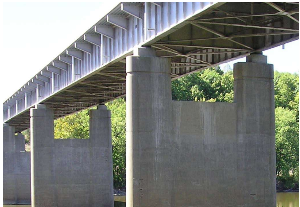
Figure 10.2.1 General View of a Deck Girder Bridge
