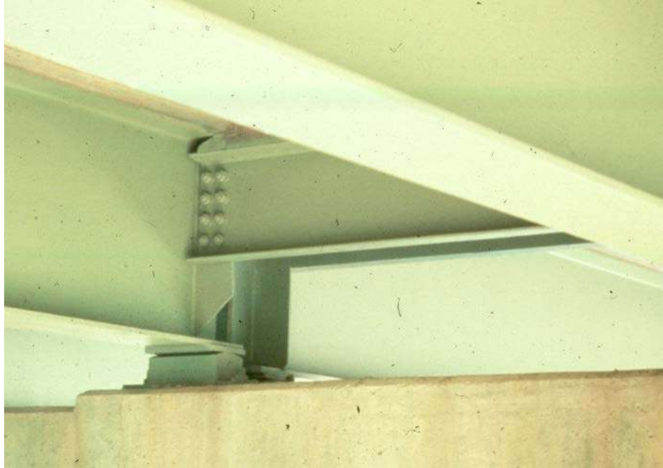
Figure 10.1.21 End Diaphragm
