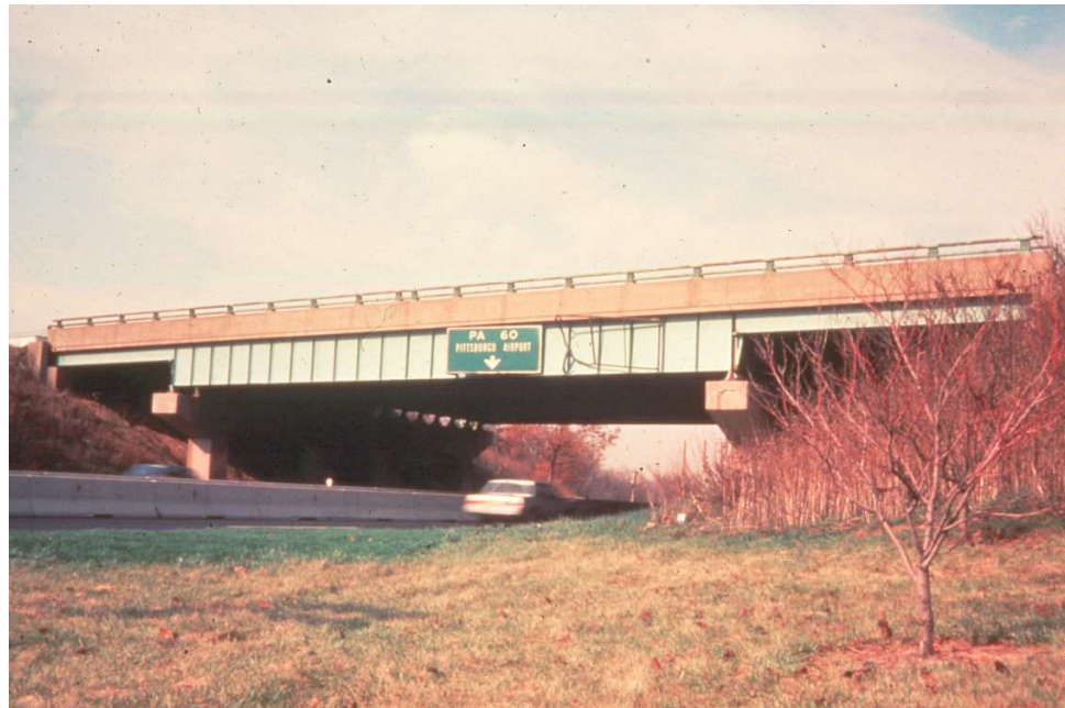
Figure 10.1.10 Combination Rolled Beams and Fabricated Girders
