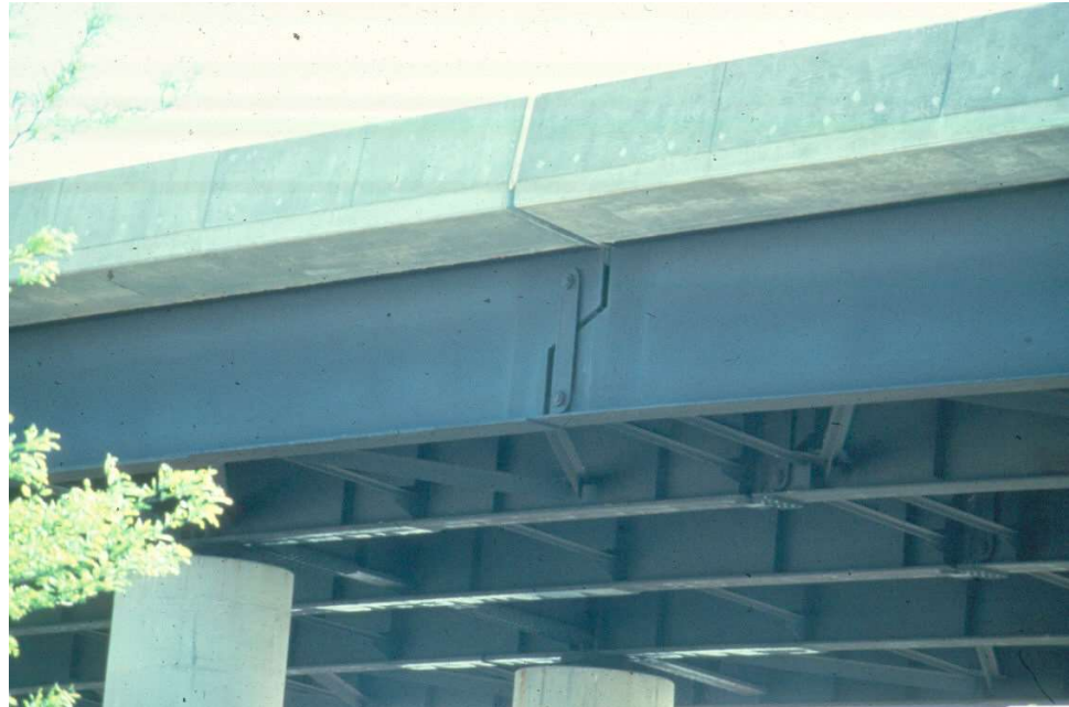
Figure 10.1.9 Fabricated Multi-girder Bridge with Pin & Hanger Connection
