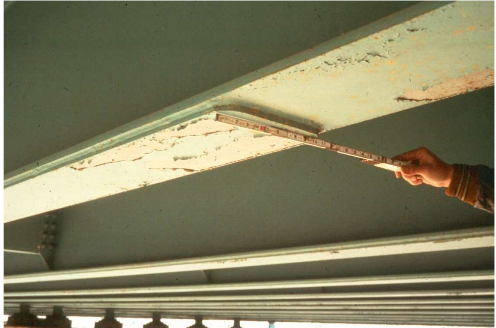
Figure 10.1.3 Rolled Multi-Beam Bridge with a Cover Plate
