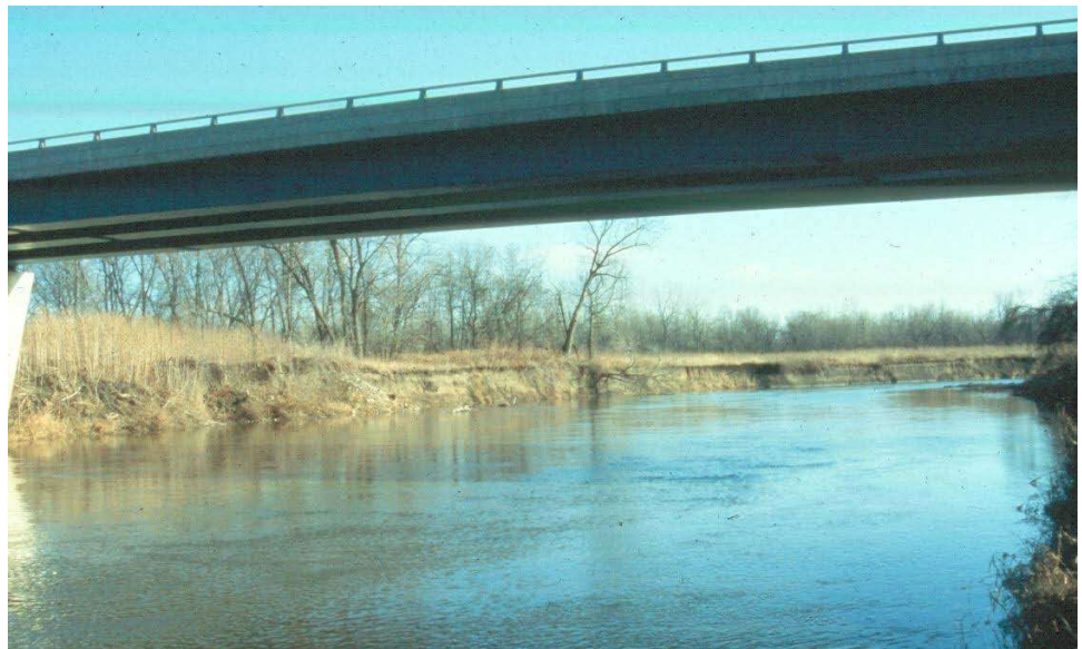
Figure 10.3.1 Simple Span Box Girder Bridge
