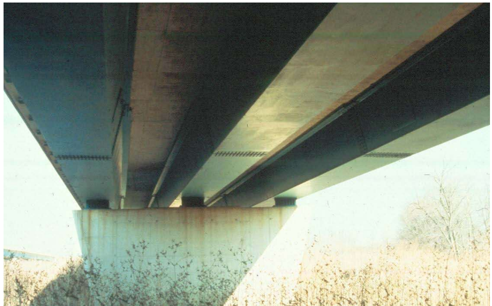
Figure 10.3.13 Redundant Box Girder Bridge
