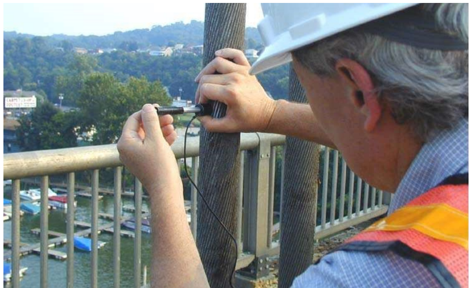
Figure 10.5.22 Performing Baseline Hardness Test on Fire Damaged Arch Cables
