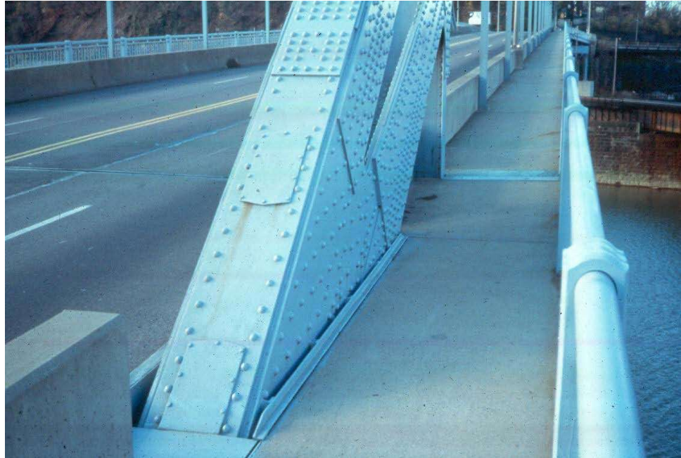
Figure 10.5.24 Through Arch Member Exposed to Traffic
