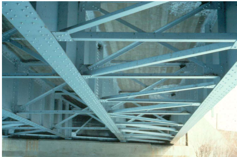
Figure 10.1.15 Straight Multi-Girder Bridge
