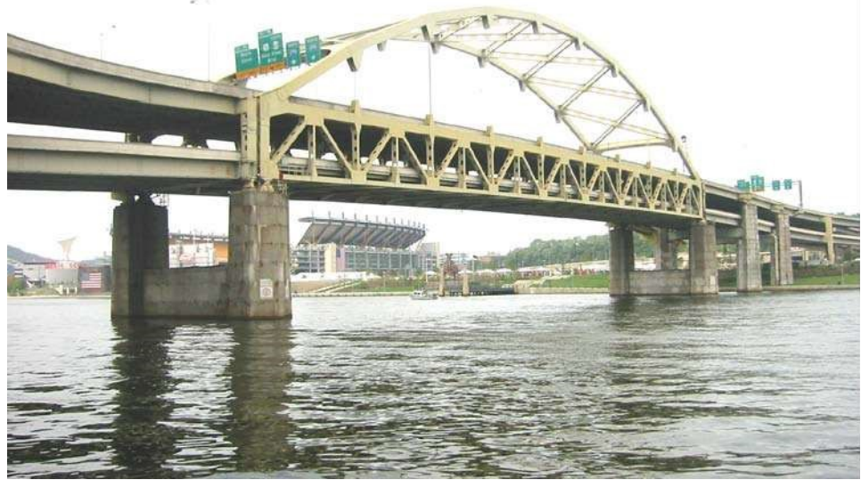
Figure 10.5.3 Tied Arch Bridge
