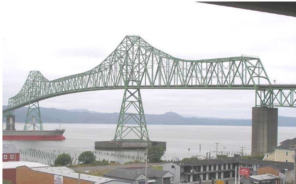
Figure 10.4.3 Through Truss
