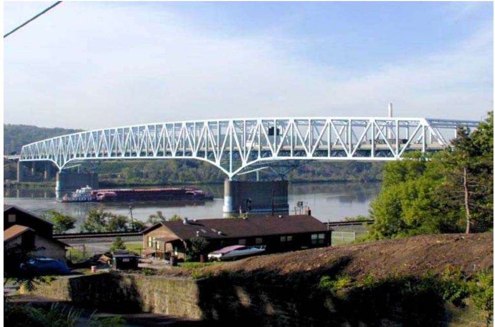
Figure 10.4.14 Continuous Through Truss
