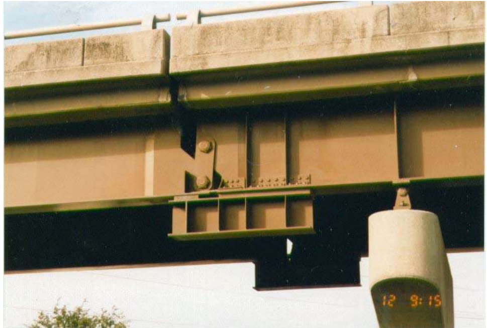
Figure 10.7.25 Underslung Catcher Retrofit
