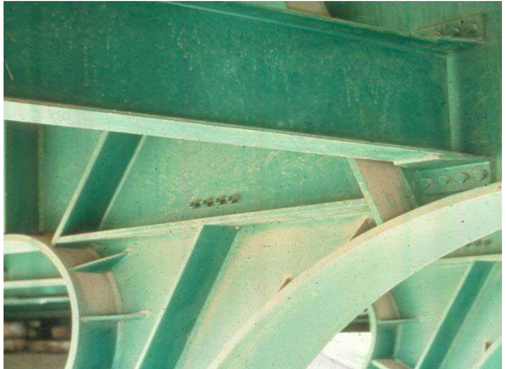
Figure 10.6.3 Connection Between Legs and Girder Portion
